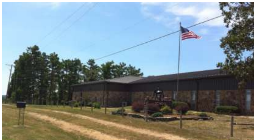
A new "pitched" roof was added to the high school in July by Noacon Inc. with funding provided by federal stimulus funds.
